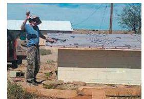
Mr. Bob working on the pump house roof.
