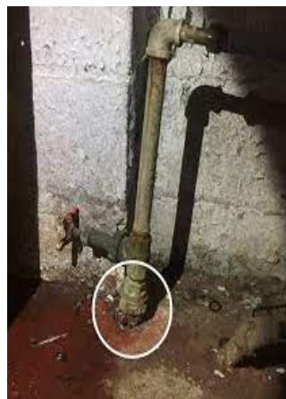
Lead Service Line – Typical solder “bulb” Characteristic at the plumbing connection “TEST AREA”
